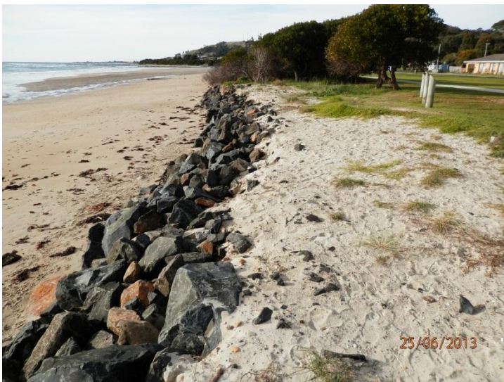
Rock revetment wall west of SLSC at playground
