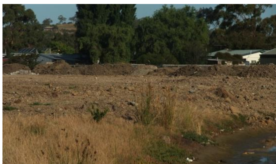
Fill to raise land levels
