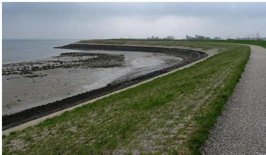
Dyke with coastal road, Holland
