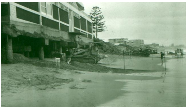
A piled coastal structure (source: WRL)
