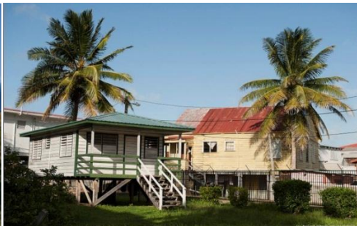
New houses elevated on piles
