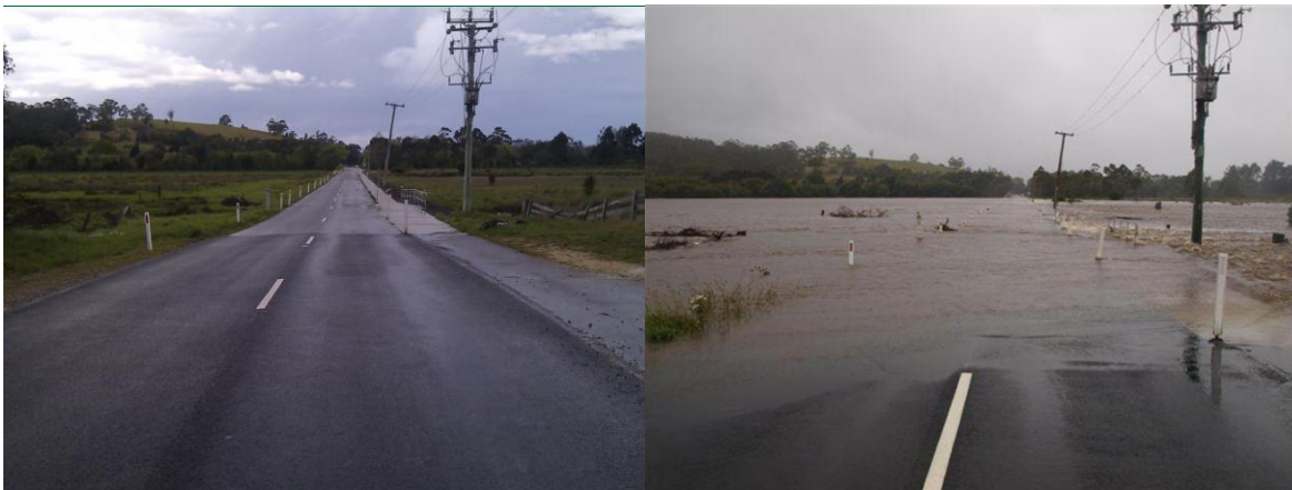
FIGURE 2 BINALONG BAY ROAD WITHOUT AND WITH FLOODING
