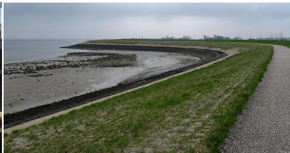
Elevated and hardened coastal road, causeway sections
