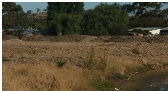
Fill to raise land levels of 'islands'
