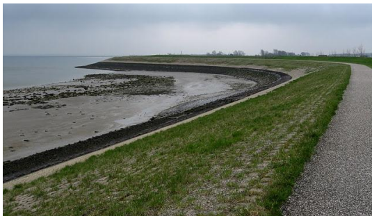
Elevated and hardened coastal road
