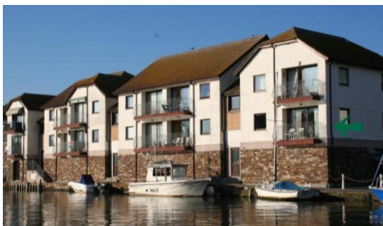
Houses elevated and designed for water levels
