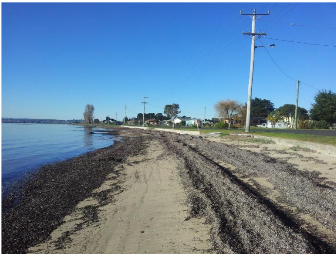
Sea wall with new sediment in front
