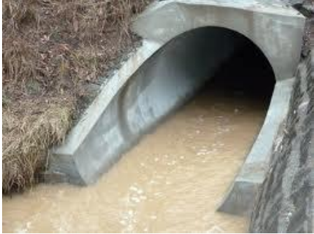
Stormwater culvert
