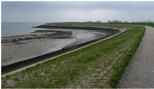
Elevated coastal road, Holland
