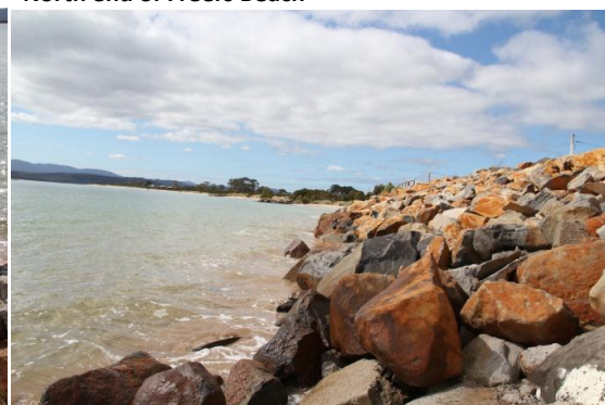
Coastal armouring at Freers Beach, north end
