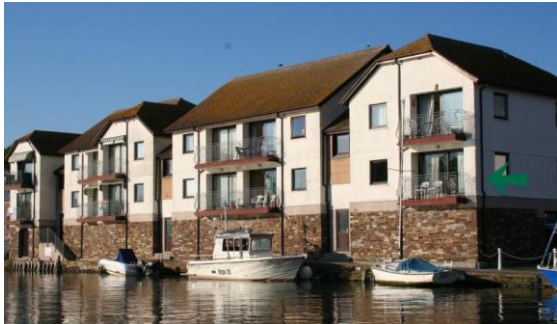
Houses elevated and designed for water levels
