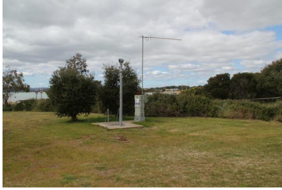
Low lying infrastructure
