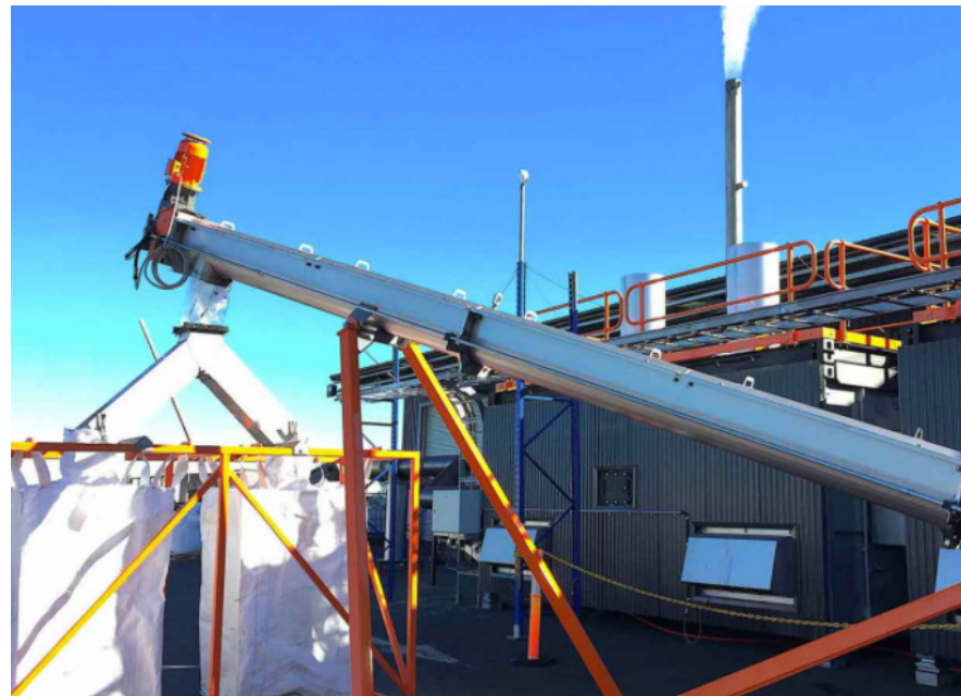
Figure 5: Logan City bio-waste plant (source: ARENA)
